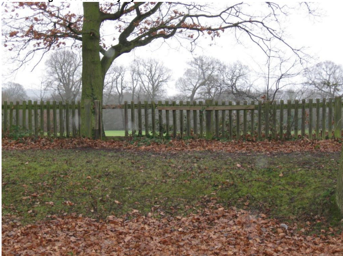
Section of the eastern part of the existing fence
